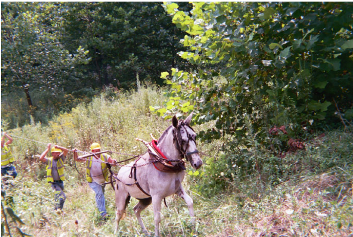
Employees of Foothills Rural Telephone Cooperative use a horse to lay fiber in rural Johnson County, Ky.
